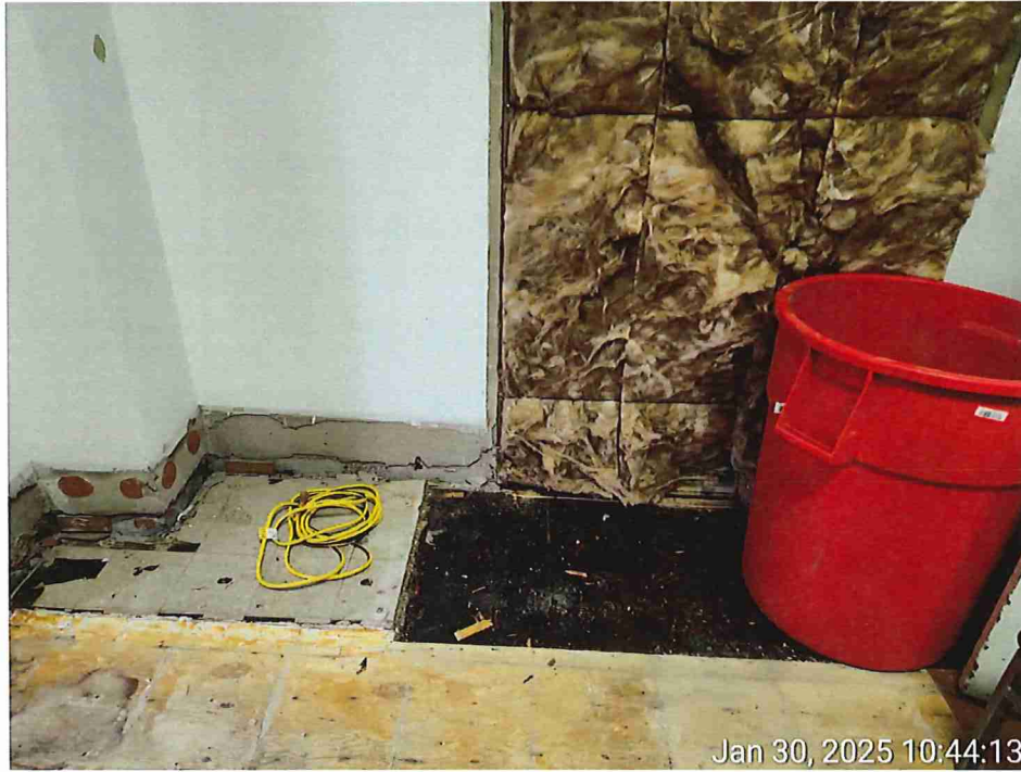
3. View of Vinyl Tile with Black Mastic
