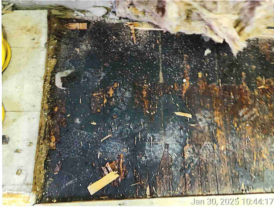
5. View of Felt Paper with Black Mastic
